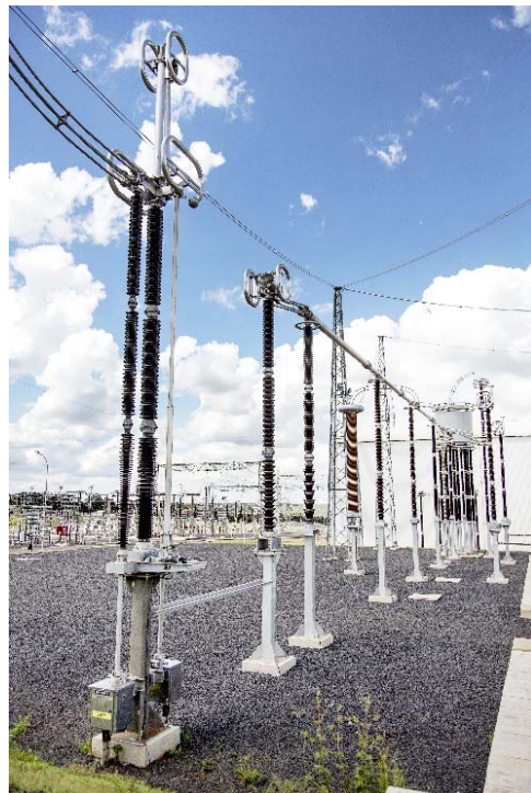
Plate 5.10 – Typical HVAC Disconnector Image: ©ABB
