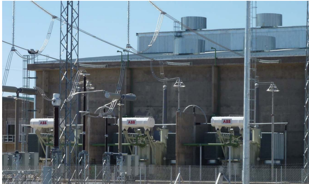
Plate 5.14 – Typical interface transformers Image: ©ABB
