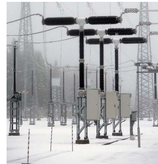
Plate 5.9 – Typical HVAC Circuit Breaker Image: ©ABB
