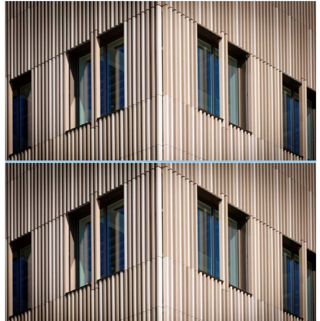
Plate 4.9 – Indicative illustrations of “baguettes”, showing shadowing effects to provide a layered texture to the facades
